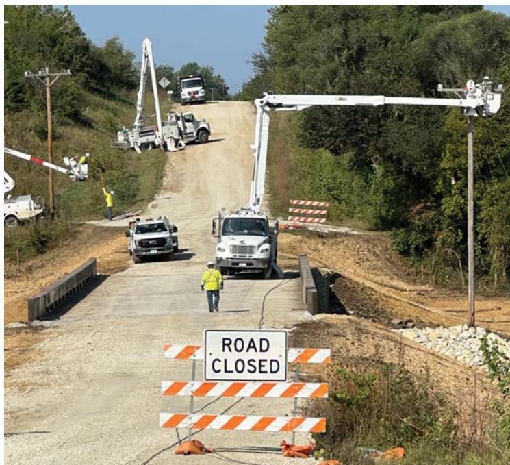
CEC crews move lines back into place following a county bridge upgrade project north of New Virginia.
