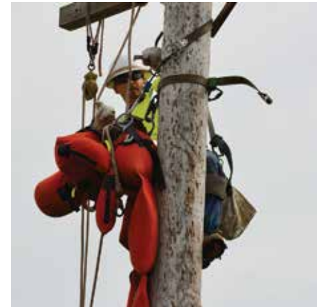
Apprentice Lineman Dom Cresta works on his pole top rescue techniques.
