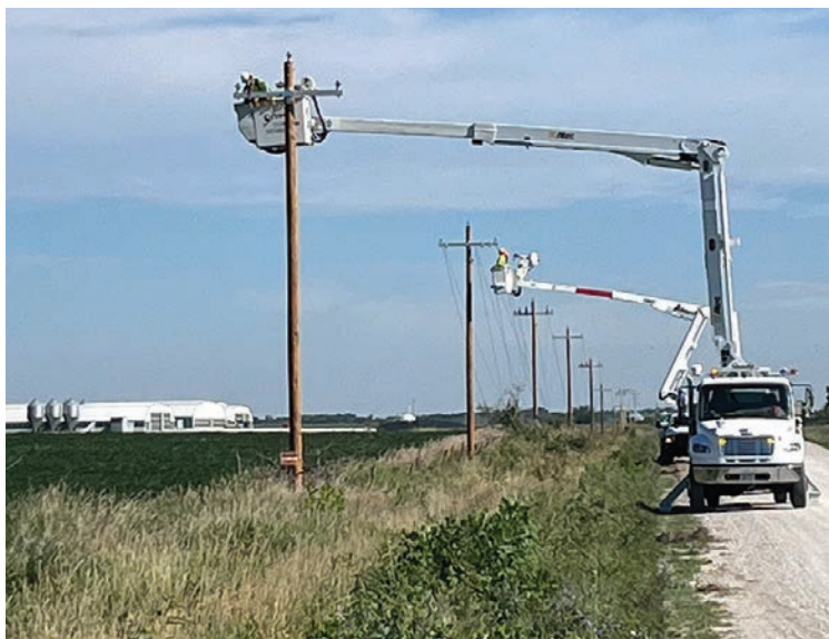
Line crews work to hang the power line conductors on each power pole prior to pulling it through to the right tension.
