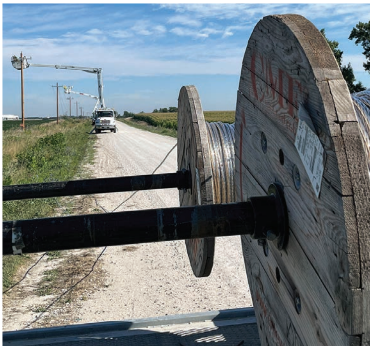
Clarke Electric linemen backstring new power line conductors onto the new three phase poles.
