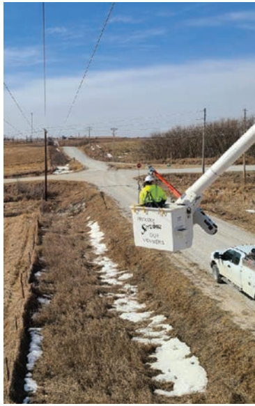
Apprentice Linemen Dom Cresta changes out a three-phase breaker bank east of the Murray substation.
