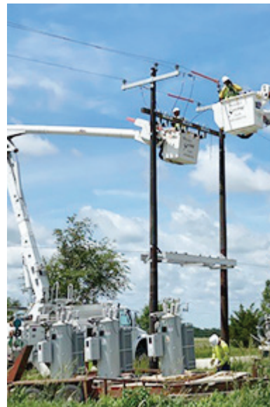
CEC crews install new 3-phase regulator banks for the Roeslein Alternative Energy project.
