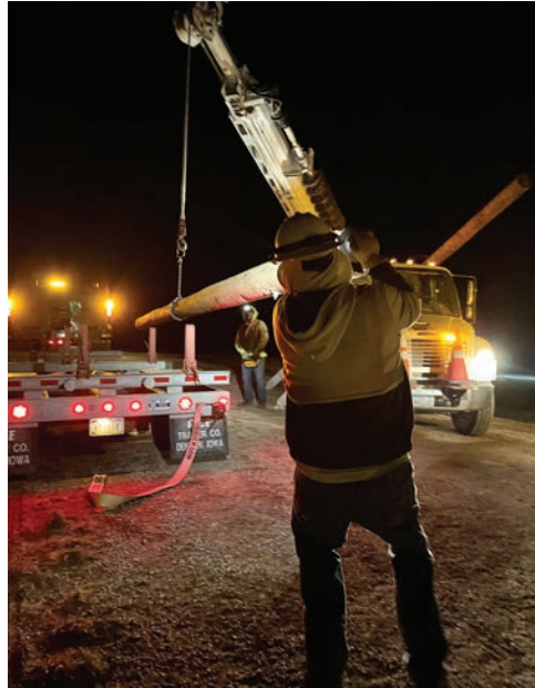
Journeyman Lineman Adam McCuddin, foreground, and Apprentice Zach Stewart, load new poles onto a truck for pole replacements during the storm.
