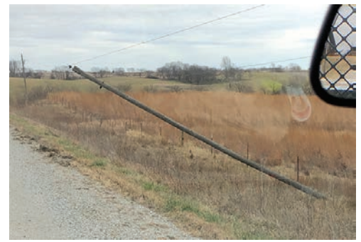
Linemen surveyed damaged poles to prioritize replacements. A pole dangerously leaning towards the road was one of many identified.
