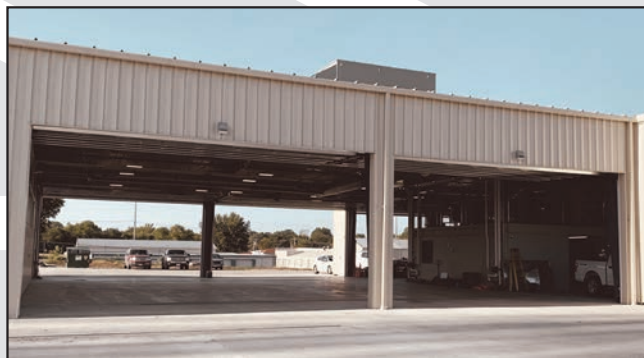
The newly expanded warehouse.
