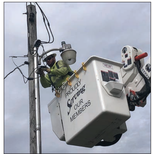
Apprentice Lineman Zach Stewart works on upgrading electric service.
